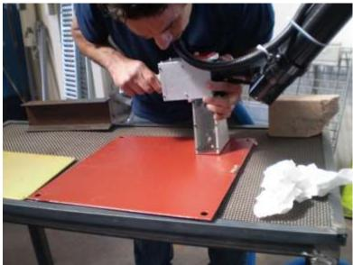
Figure 5-5. Laser Stripping Copper Paint Panel
